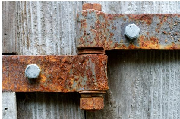
Please check **hinge condition**. Any rust and dirt will reduce the effectiveness of gate closer. Please clean and lubricate the turning point of the hinge.
